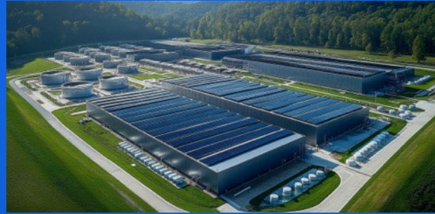
Hyperscale data center design Site-specific planning and design for LEED Gold certified facility
