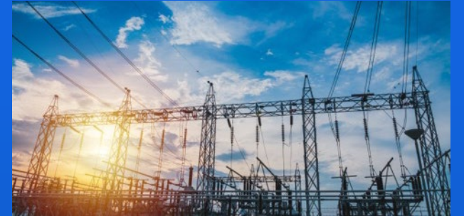
Substation construction Substation to solve fast expansion needs
